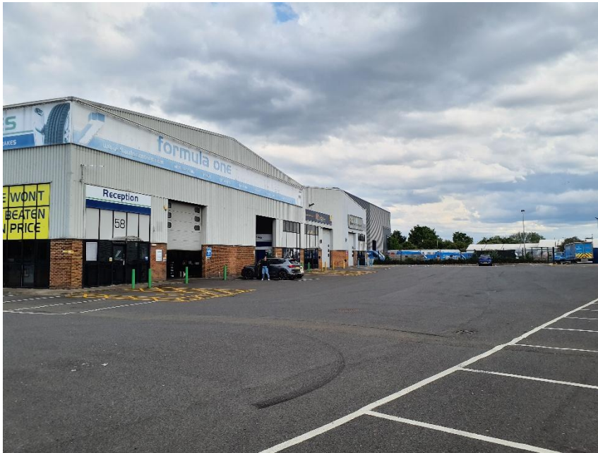
Figure 1.4: Typical commercial / industrial units on Mill Way, Sittingbourne.
