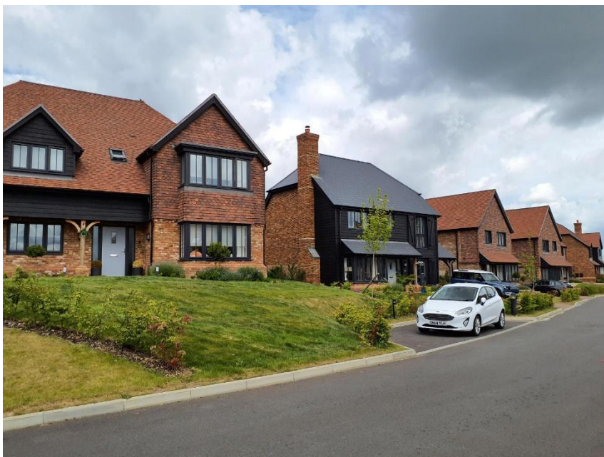
Figure 1.3: Typical recent residential development on Hill Farm View at Keycol.
